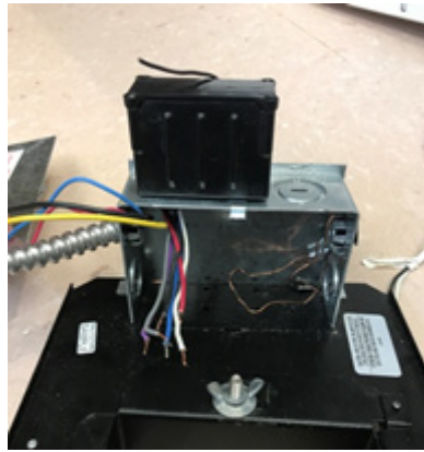
Figure F: LVDC Luminaire Controller (ESCD1000) attached to the junction box and fastened with supplied locknut
